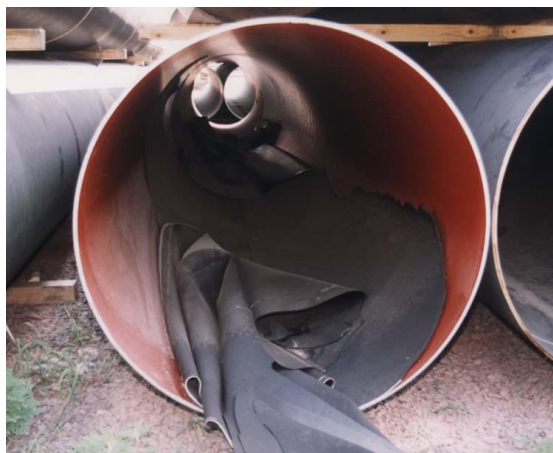
Figure 2. The failure of an elastomeric polyurethane lining
